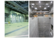
2 Platform and combustible waste pit
